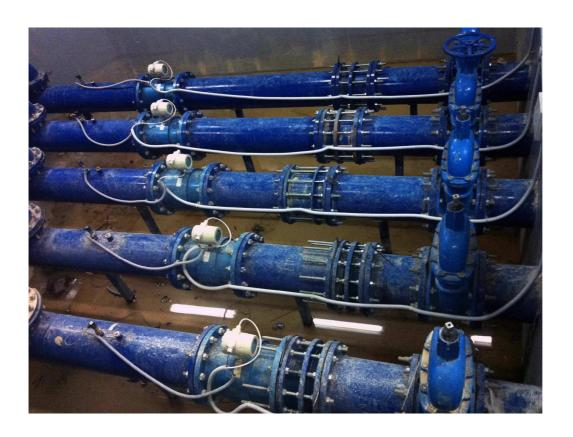
**EGYPT - El Ayat Water Treatment plant** We installed 6 EMF sizes DN300 to DN1200
