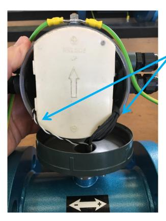
Place the battery as showed in the picture. The cable of the electrode must be on one side of the pack and the cable of the coils on the opposite side
